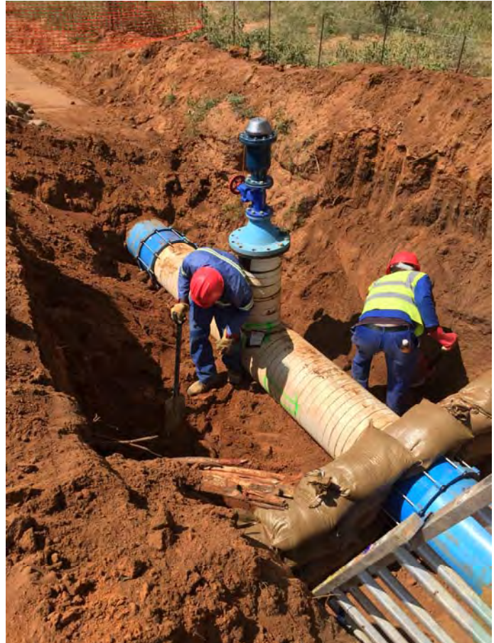
Section of 13 km pipeline
