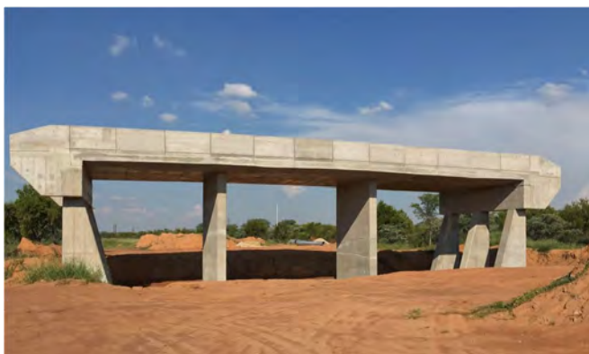
Completed bridge on the rail link
