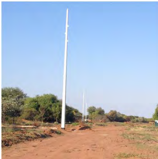
132kV powerline construction
