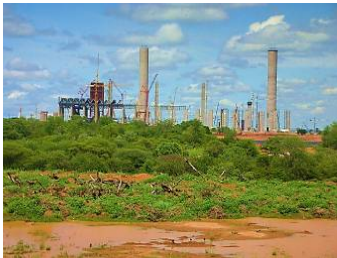
Figure 8. Medupi Power Station under Construction
