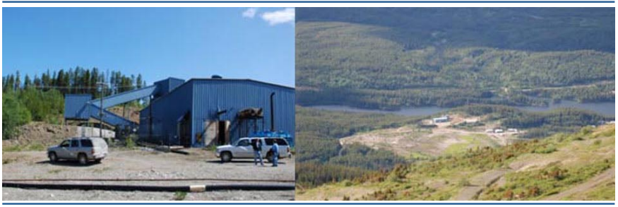
Figure: 270 tpd Mill Facility (left); Mine and Mill Site (right)
