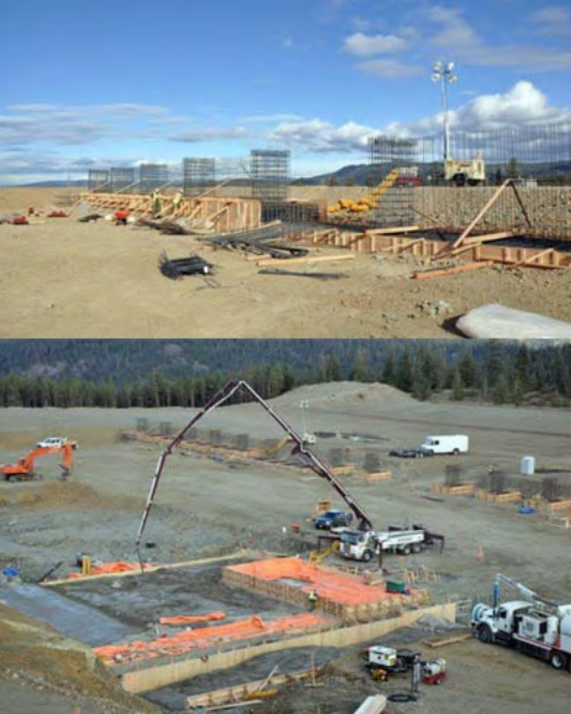
Figure: Building of Concentrator Foundations
