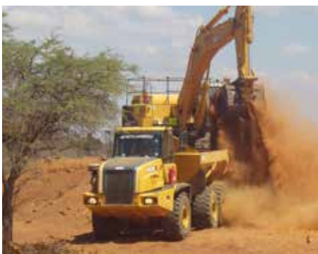
Beginning of the construction camp ground works.
