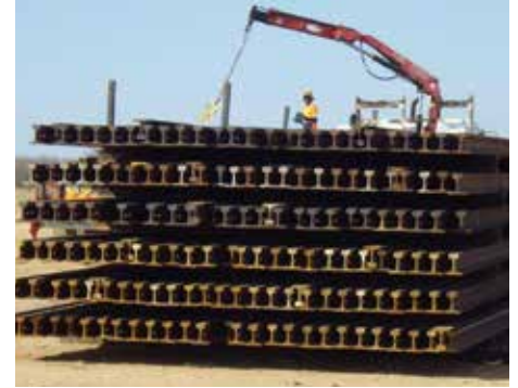
Railway tracks ready for construction of the rail loop.
