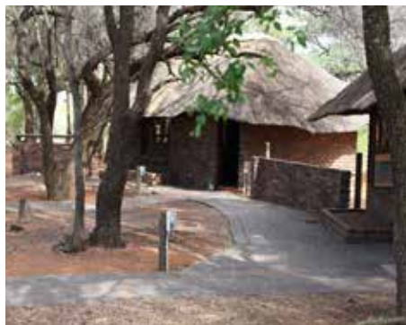
Accommodation being renovated.
