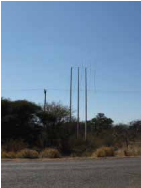
Powerline poles at installed at 13 locations along the Boikarabelo rail route allowing safe construction and passage.
