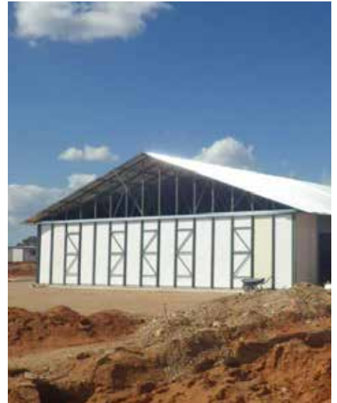
Dining Room construction
