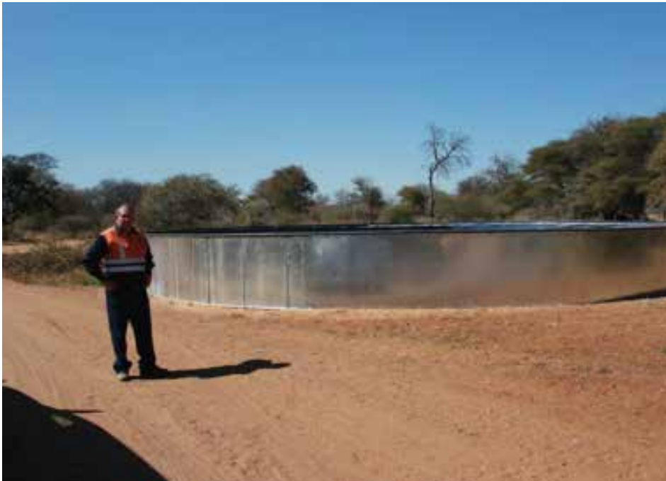
The 27,000 litre “Staalboer steel panel dam” installed at Bitterfontein.
