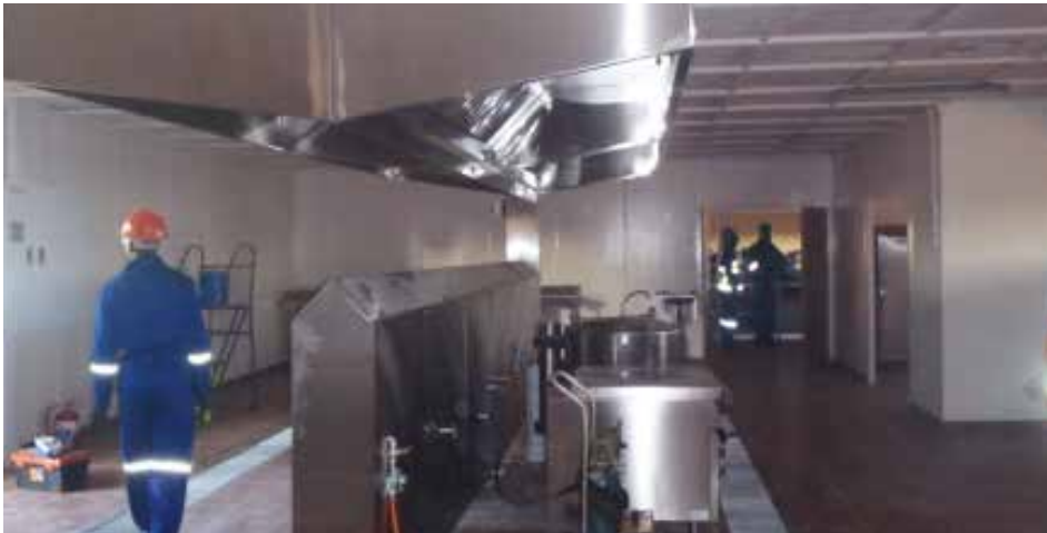
Finishing touches being put to the kitchen and dining room.
