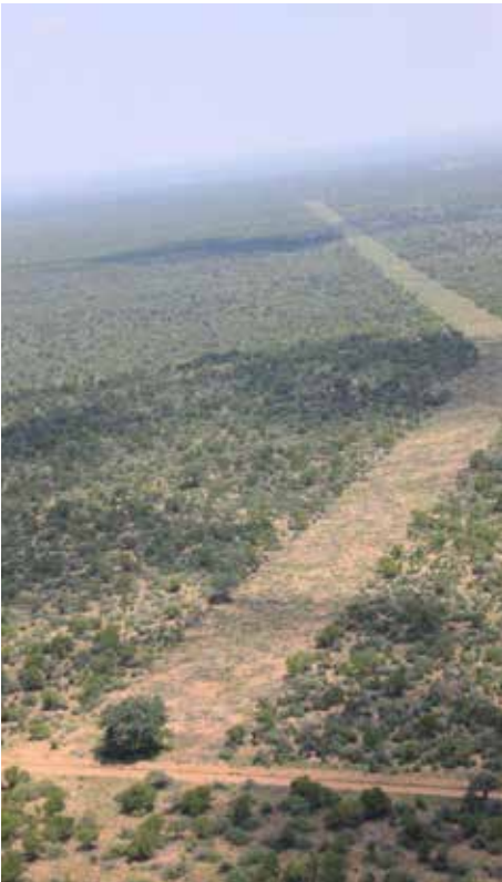
Rail line cleared on Bitterfontein southern boundary.
