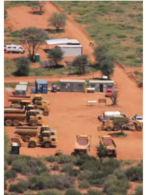
Temporary construction office area for Protech Khuthele.
