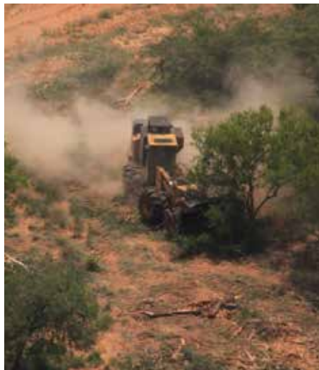
Lenco bush clearer at work along the rail line.
