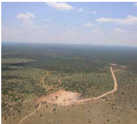
Borrow pits on Witkopje for the terrace construction material.
