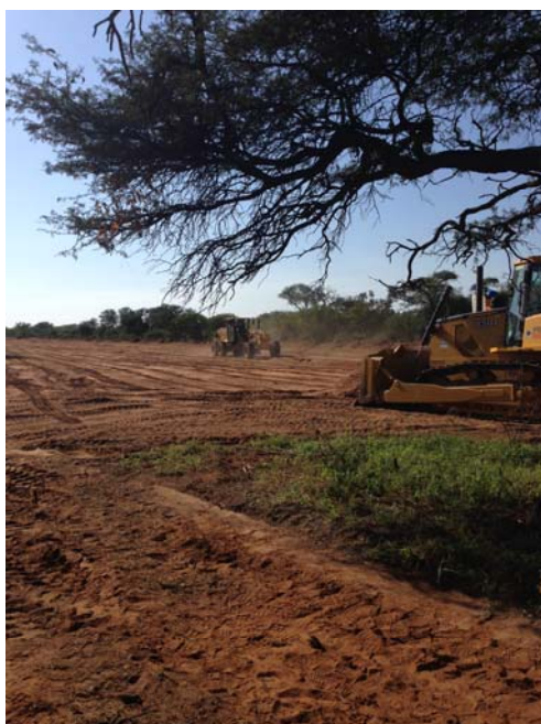
Rail line earthworks
