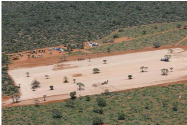
Earthworks at construction camp
