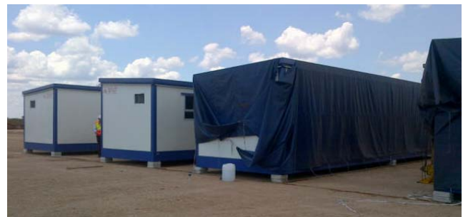
Initial construction camp units delivered to site
