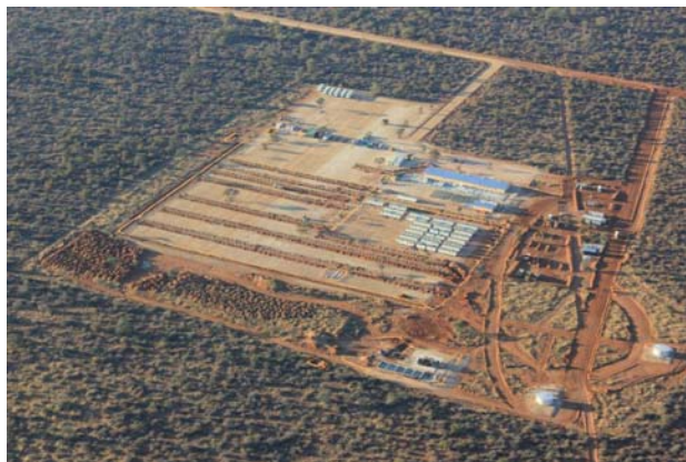
The construction camp
