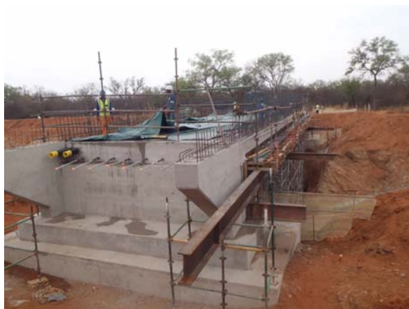
Bridge construction on the rail link
