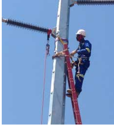
Conco employee installing conductors on the 132KV line.
