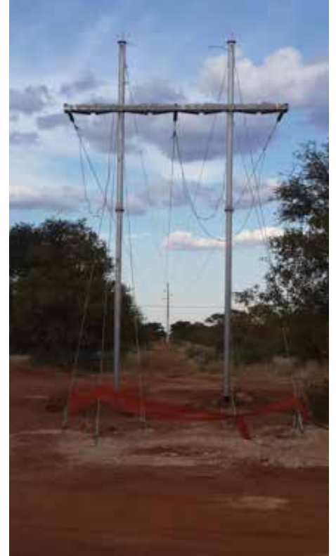
An illustration of the stringing progress at the end tower before dropping down to the main in-come sub-station.
