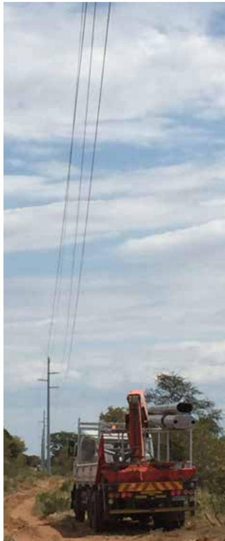
An illustration of the stringing progress at the end tower before dropping down to the main in-come sub-station.
