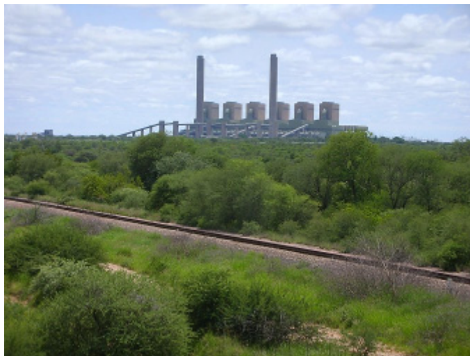
Figure 7. Matimba Power Station
