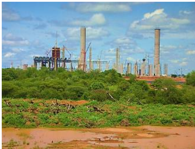
Figure 8. Medupi Power Station under Construction
