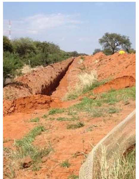
13 km pipeline trench
