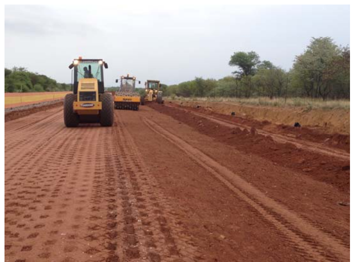
Network Stabilisation Facility
