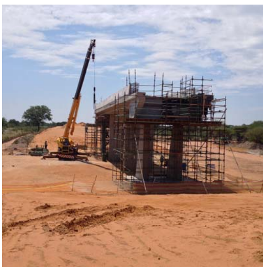
Bridge construction on the rail link
