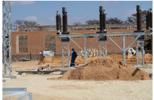
Switch Room Construction in Background
