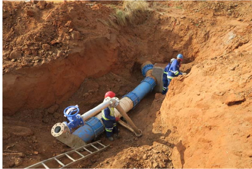
Section of 13 km pipeline
