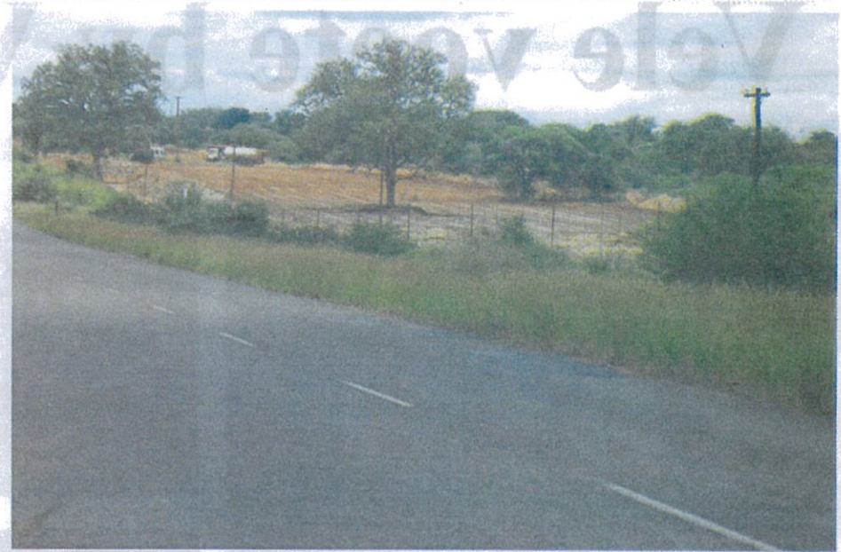
Preparations for the railway line next to the Steenbokpan Road are in progress
